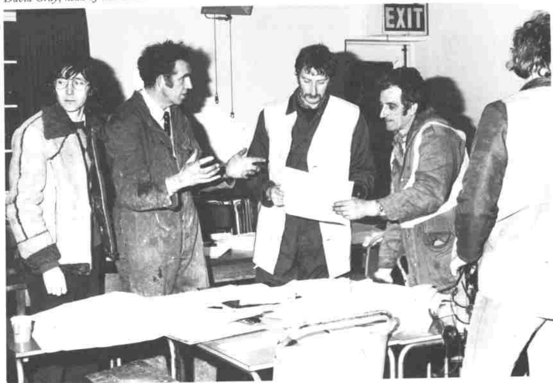
Bernard Hatch briefing men on cable laying operations
