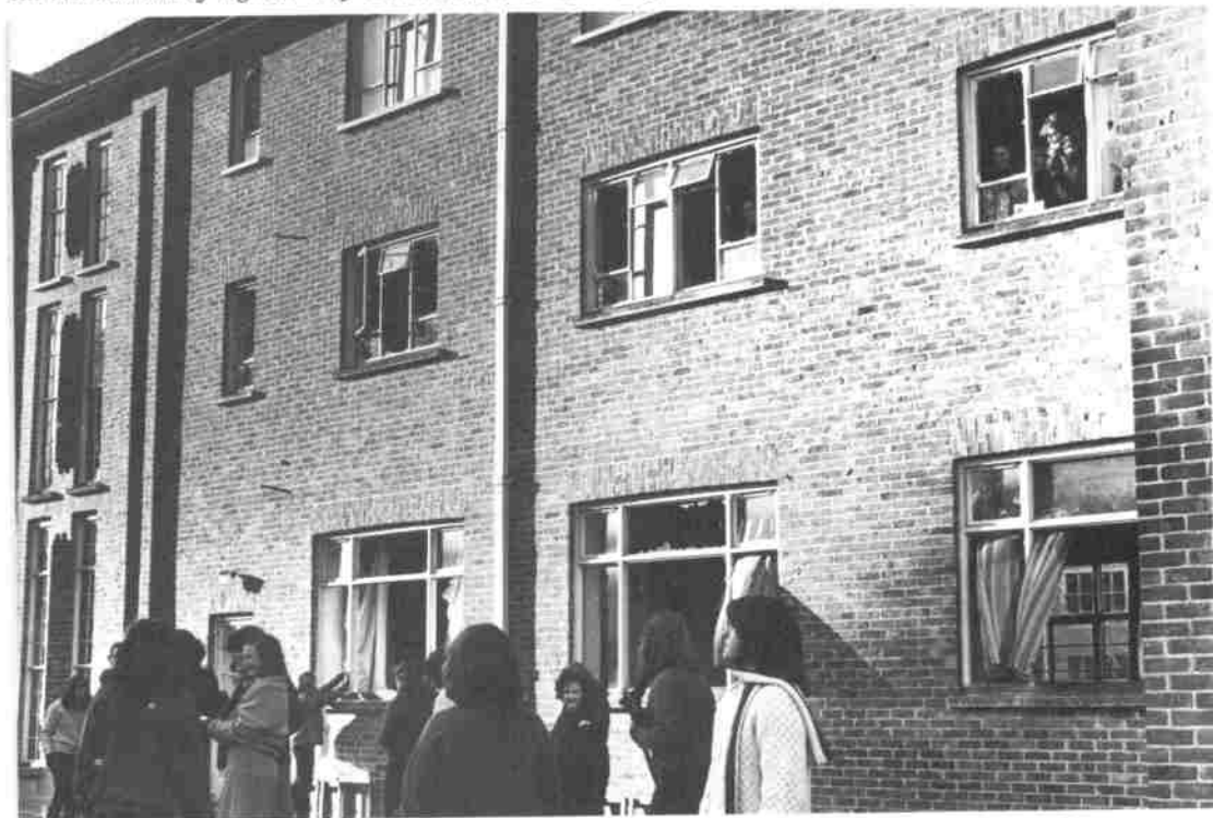
Broken windows in St Gabriel's House, St Leonards-Mayfield Convent. St Gabriel's overlooks the former exchange
