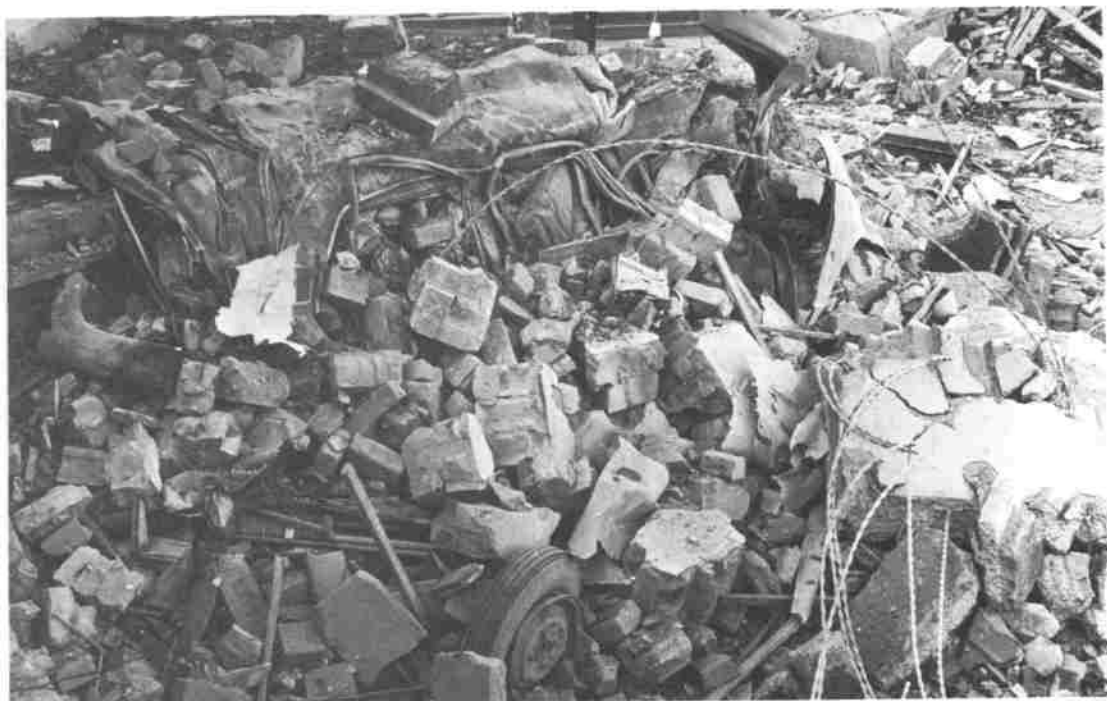
All that remained of engineer Tony Burton's car. Note the wellington boot on the left hand side
